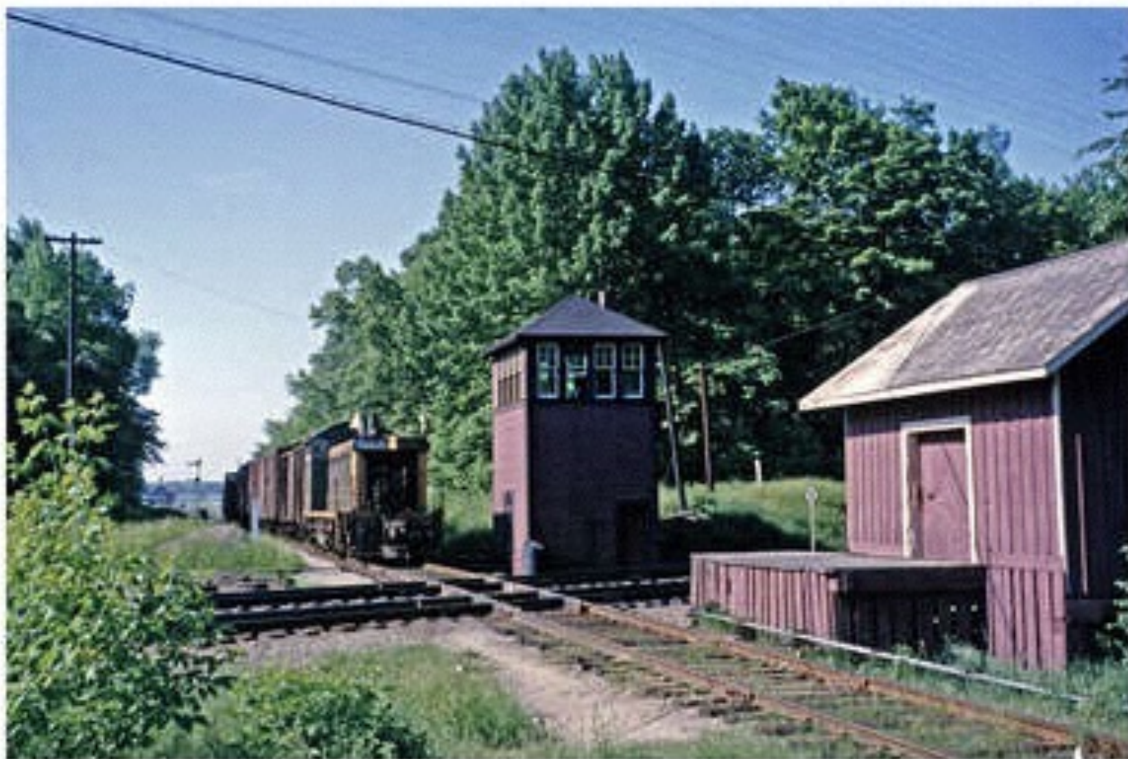
The CNR's daily except Sunday wayfreight has departed Milton station in the distance and is about to cross the double-tracked CPR Toronto to London mainline on June 6, 1959. This train operated from Hamilton to Allandale via Milton, Georgetown, Inglewood and Caledon. The signals protecting this crossing were manually operated with long rods stretching from the signal to huge levers located upstairs in the interlocking tower and required much strength to move.
